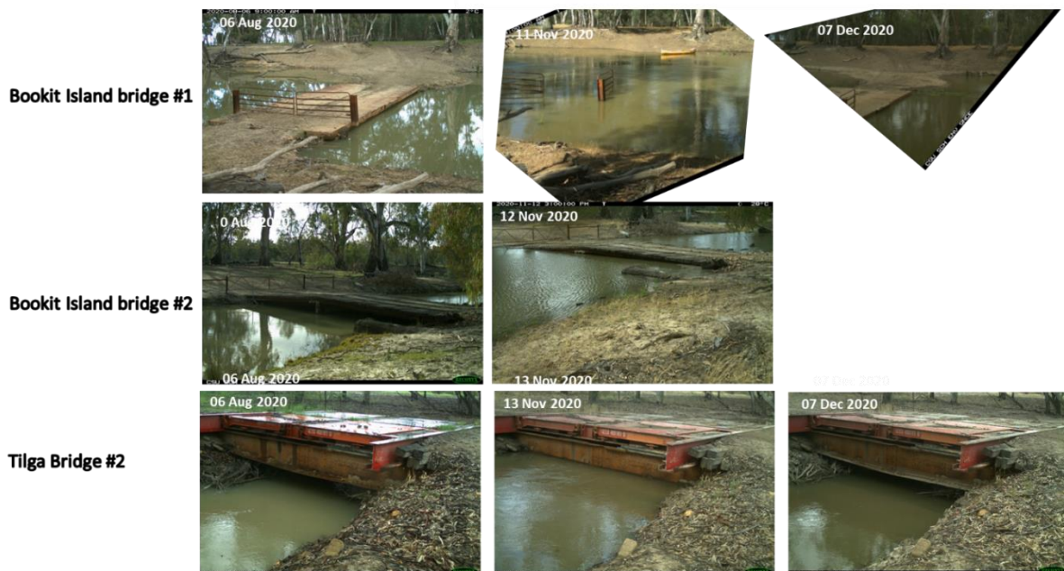
Figure 4.8 Changes in water level near three bridges during the 800 ML/d flow trial in 2020. The camera installed at Bookit Island Bridge was knocked by stock and so the photo points were taken on angle for part of the flow trial.
