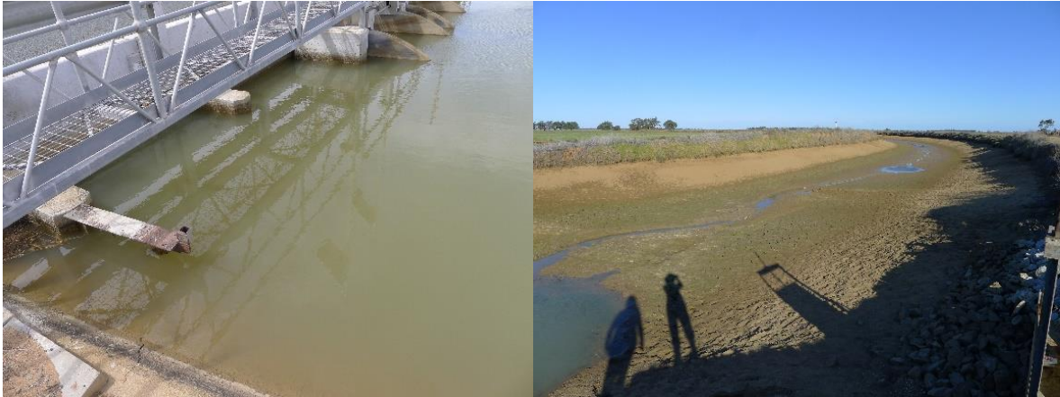
Figure 5.4 Mulwala Canal in March 2022 (left) and July 2021 (right). (Photo: Xiaoying Liu)
