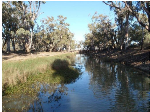
Merran Creek Bridge, Merran Creek
