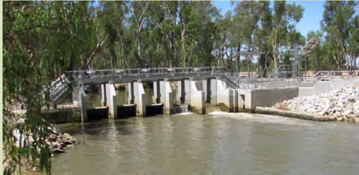
Weir at the regulator on Yallakool Creek (Photo: Robyn Watts)
