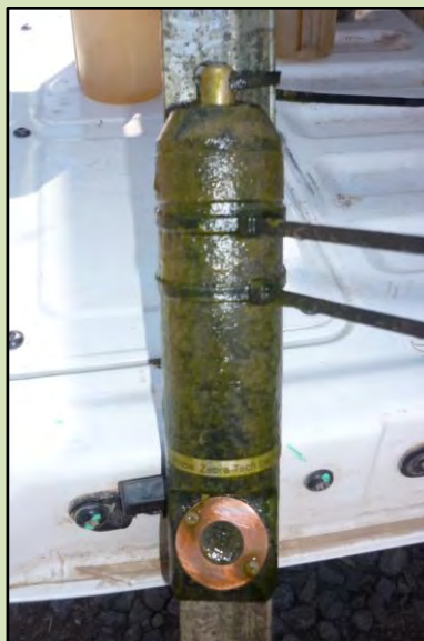
A high level of biofilm growth impacted the performance of the dissolved oxygen probe in zone 2 (no environmental water) and required additional maintenance. Photo: J. Abell
